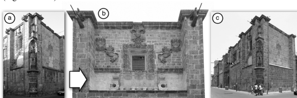
Figure 1. a) Church before restoration. b) Area where architectural elements were discovered (arrow) that include three niches for the placement of religious sculptures. c) Church after restoration.
